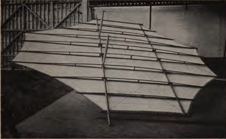
Fig. 76.—The forward rudder of my large machine, showing the fabric attached to the lower side. The top was also covered with fabric. This rudder considered as an aeroplane had a very high efficiency and worked very well indeed.
